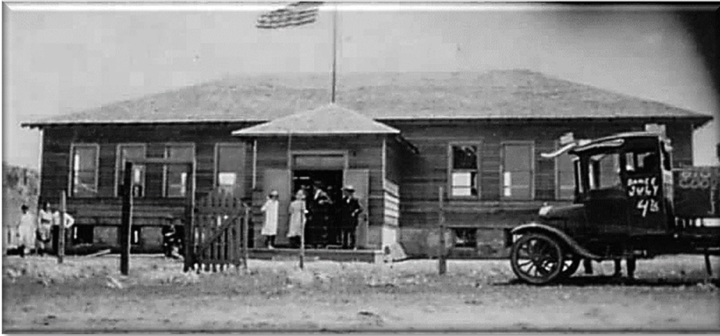
Original Lepper Memorial Hall. Source: Flatwillow Vertical File, Petroleum Co.
