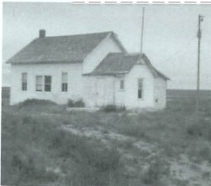
"The power was disconnected in September 1987 and the doors were locked on the Blakeslee schoolhouse."
