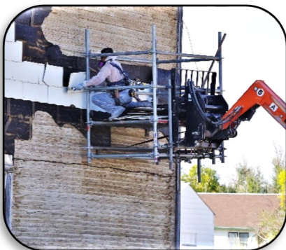
Abatement of asbestos & lead in the Odd Fellows Hall. Photo Credit: Ralph T. Corbett
