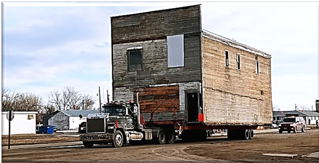
The Odd Fellows building being moved down main street to its new location Feb. 7 th . Photo Credit: Laura Nowlin
